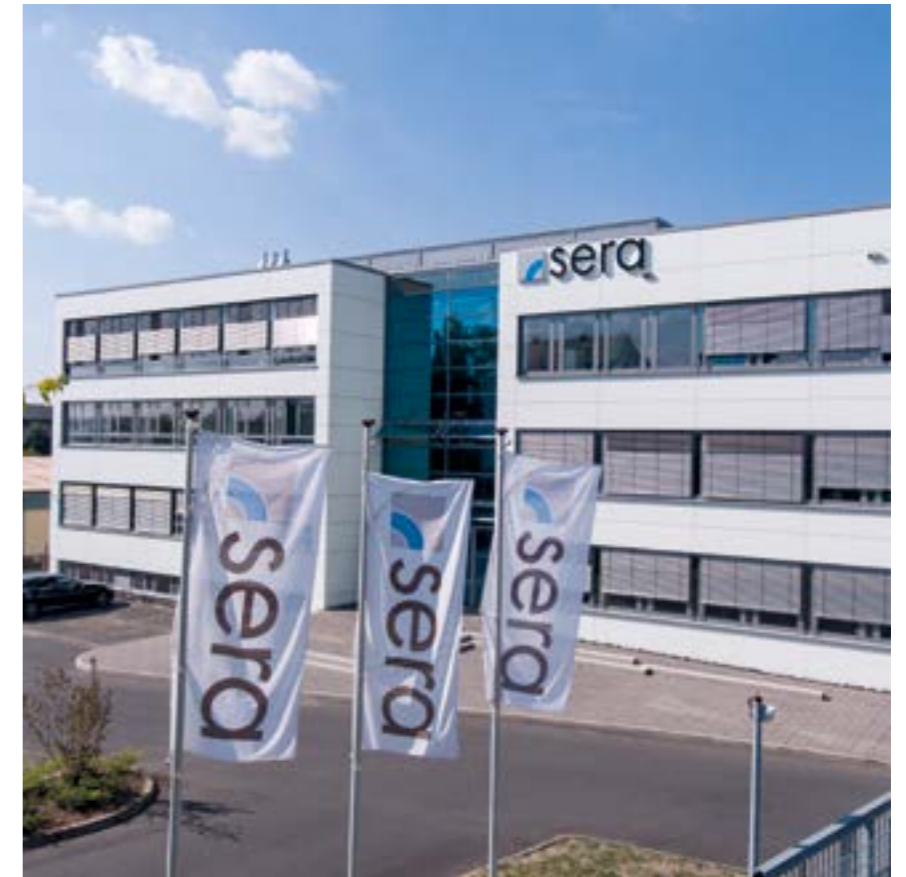
Das sera Headquarter in Immenhausen.
