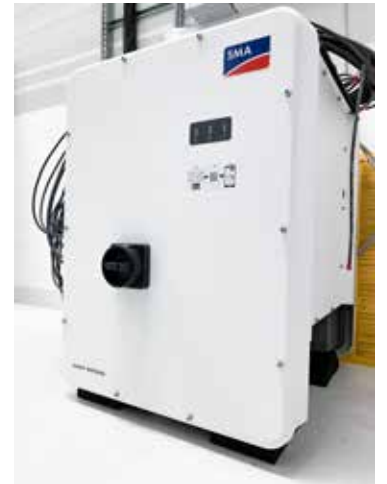
View of the main site with part of the new photovoltaic system on hall 4, PV inverter for converting the direct current into alternating current
