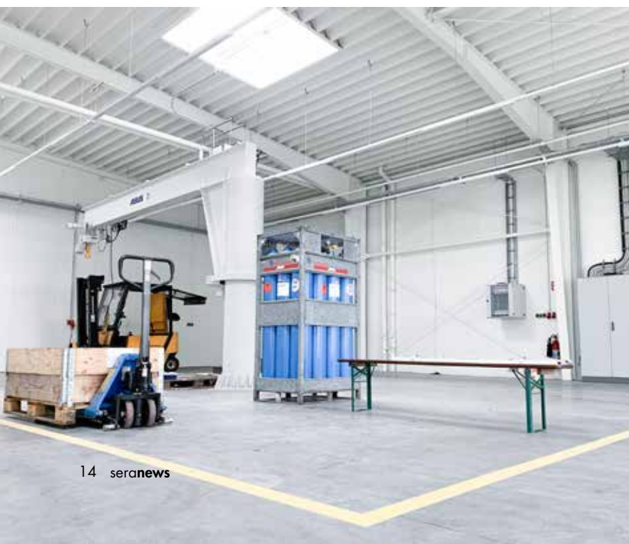
Renovated Hall 6 with new technology and larger skylights for more brightness
