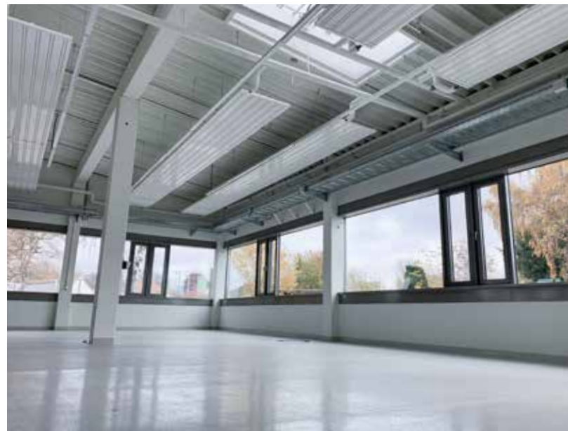
View into the newly designed Hall 4 with transparent glass front to the outside
