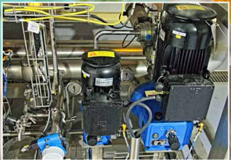
sera multi-layer diaphragm pumps ensure precise dosing in a system from our partner Centec
