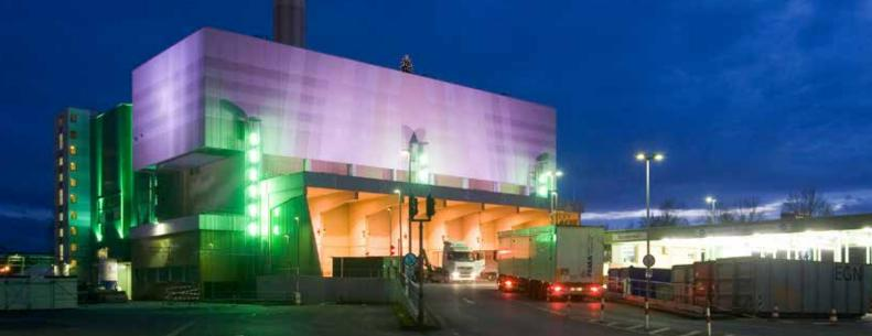
Recycling of the waste from Bonn and the surrounding region is carried out by Müllverwertungsanlage Bonn GmbH (MVA), a subsidiary of Stadtwerke Bonn (Bonn Public Utilities). Over 1,000 tonnes of waste, which has to be disposed of in a safe and environmentally friendly way, is delivered to it every working day. In a complex thermal process, the waste is first incinerated and then processed. Flue gases are created when the refuse is burnt.
