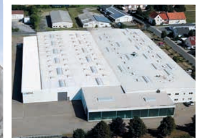
2016 – Construction of factory location 2 at the Immenhausen site (Germany).
